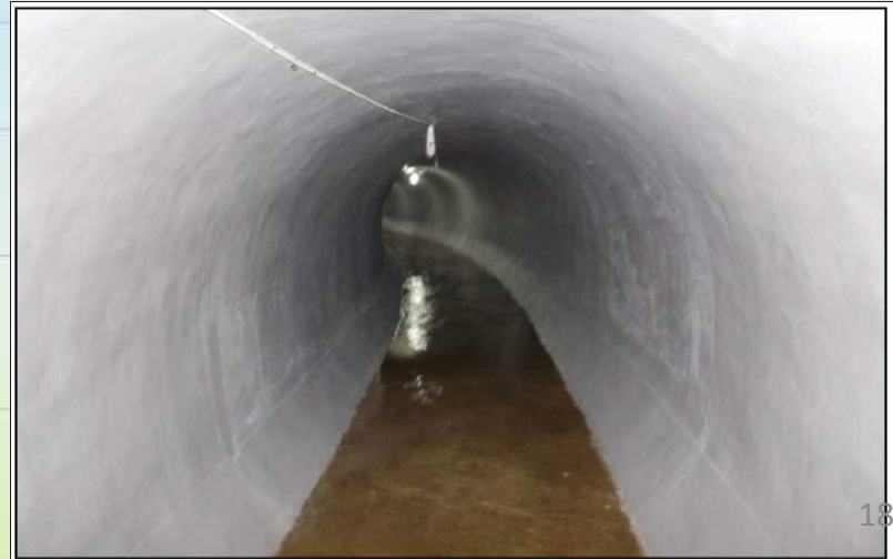
Repair work of Ngalaik Dam Outlet Conduit Barrel
