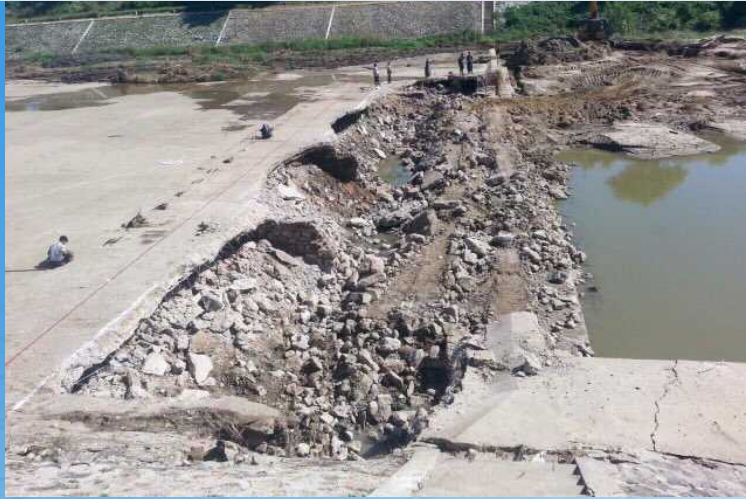
Repair work of Ngalaik Dam Outlet Conduit Barrel
