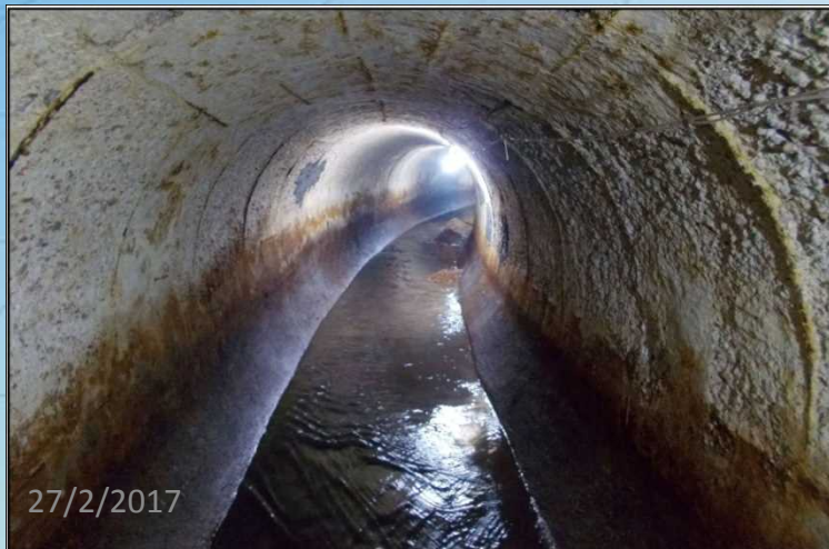
Repair work of Ngalaik Dam Outlet Conduit Barrel
