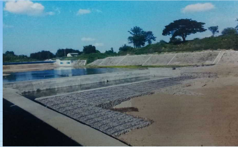
Repair work of Ngalaik Dam Outlet Conduit Barrel
